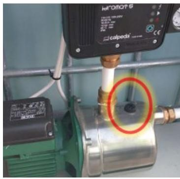
Where a Stuart Turner Boostamatic water pump is fitted and the supplying water tank runs low, and is then filled up again, it is possible that this will introduce air into the pipework.
