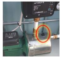
Where a Stuart Turner Boostamatic water pump is fitted and the supplying water tank runs low, and is then filled up again, it is possible that this will introduce air into the pipework.
